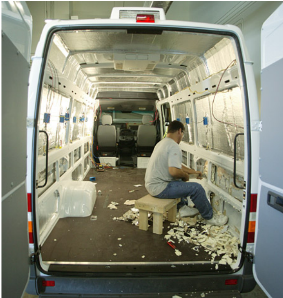
Figure 17-21. Installing insulation during initial conversion of the Suspended Animation Sprinter van.
