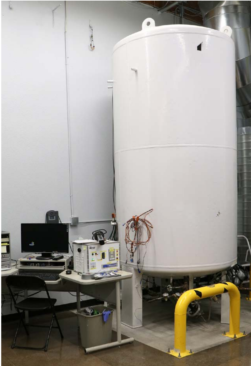
Figure 20-18. The bulk storage tank for liquid nitrogen in Alcor's patient care bay. Its capacity is 900 gallons.
