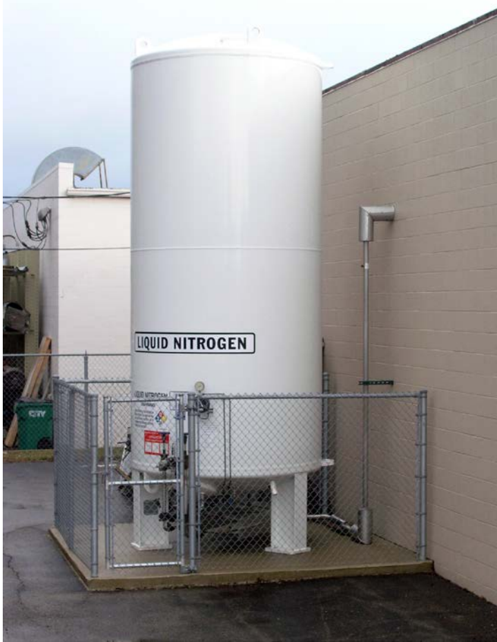
Figure 20-30. The 3,000-gallon bulk storage tank outside the Cryonics Institute.
