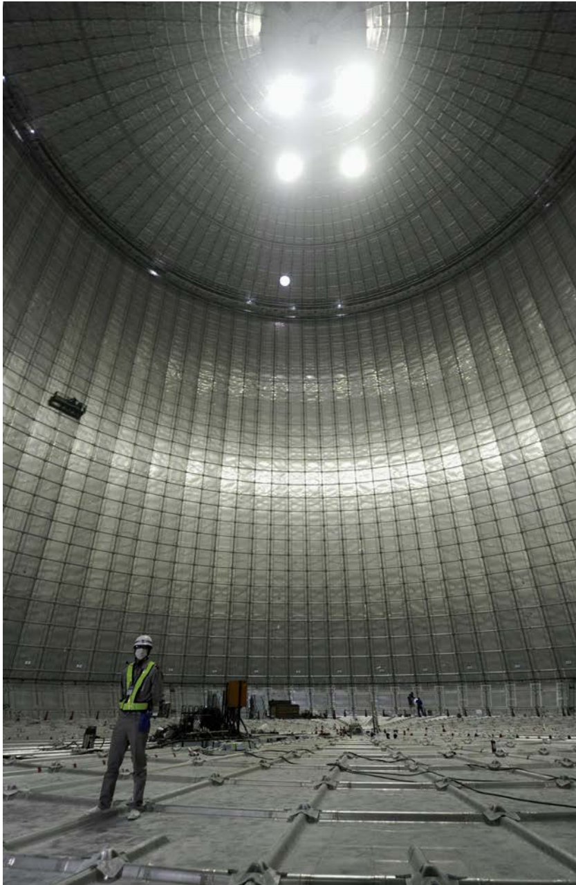
Figure 20-38. A 250,000-kiloliter liquefied natural gas storage facility under construction in Yokohama.
