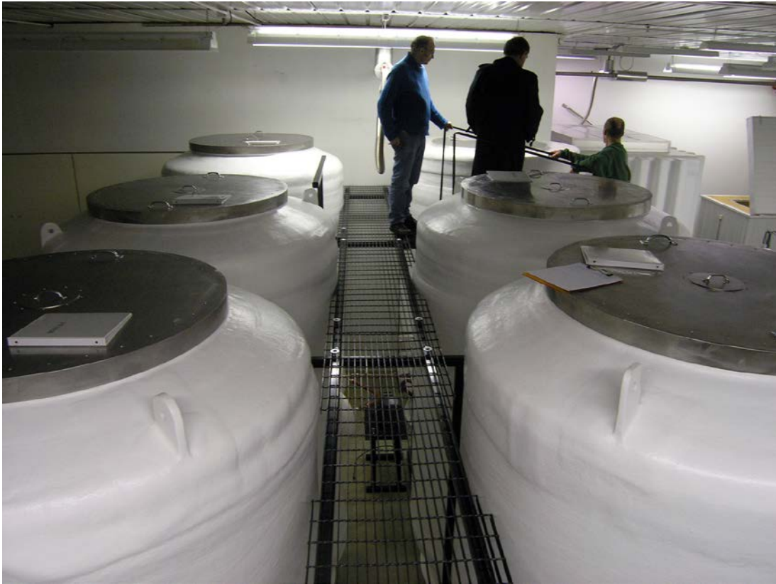
Figure 20-28. A catwalk allows access to the lids of the cryostats at the Cryonics Institute.
