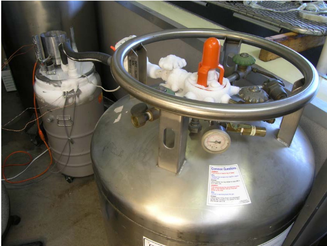
Figure 19-3. The storage dewar in the foreground is supplying liquid nitrogen to the neuro cooldown dewar in the background.
