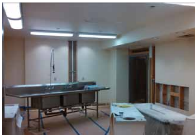
The operating room under construction.
