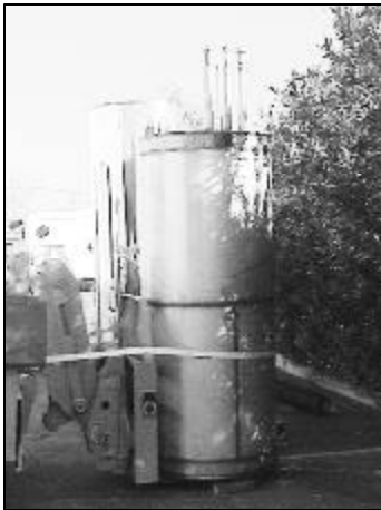
The pressure vessel, in its lifting harness here, awaits placement in bigfoot 1, behind it.
